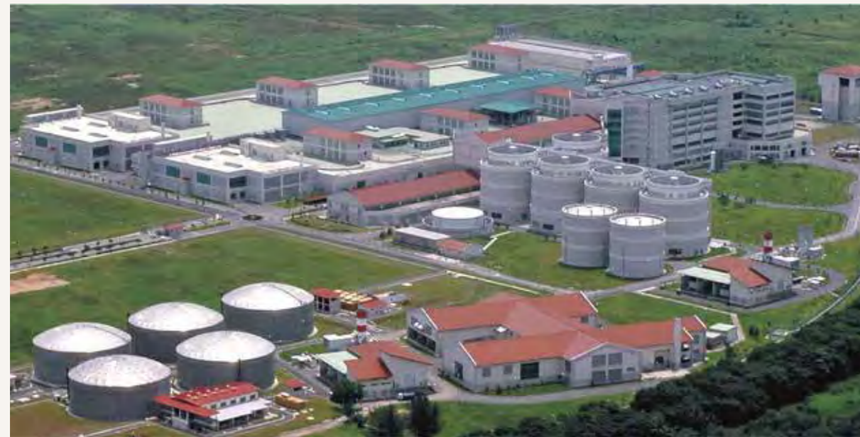
The biogas produced in the digesters at Changi Water Reclamation Plant (above) is used as fuel to either generate electricity to power the operation of the treatment facilities or dry dewatered sludge further to become dried sludge.
