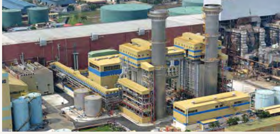
A natural gas-fired combined cycle plant converted from a conventional oil-fired steam power plant
