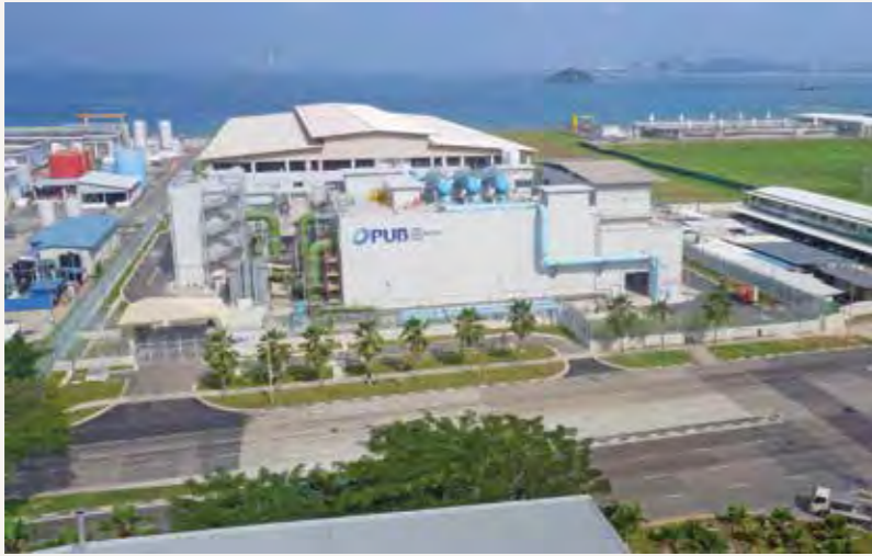
The seawater reverse osmosis membrane vessels used in the desalination plant are more energy-intensive compared to treating water from the local catchment.
