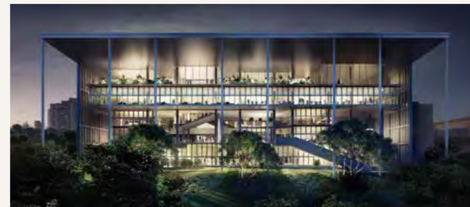
NUS School of Design & Environment, winner of the Green Mark Award for Buildings – Zero Energy Building 2019
