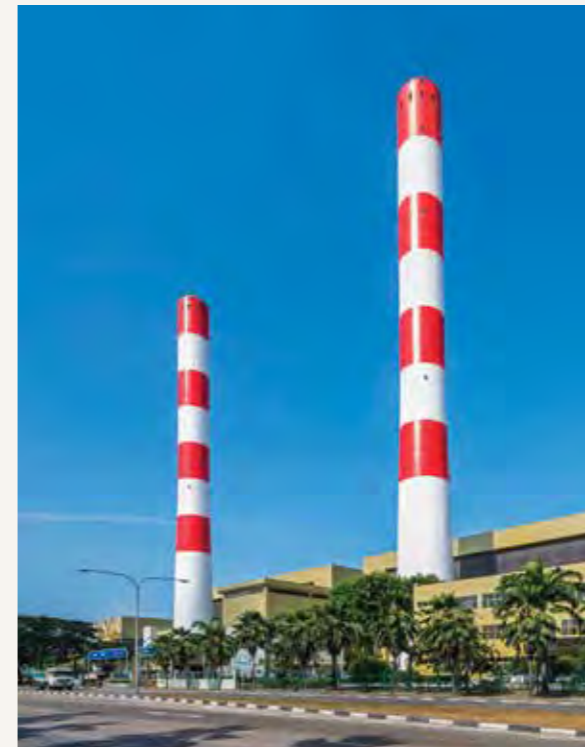
Tuas South Incineration Plant, one of the waste-to-energy (WTE) plants in Singapore
